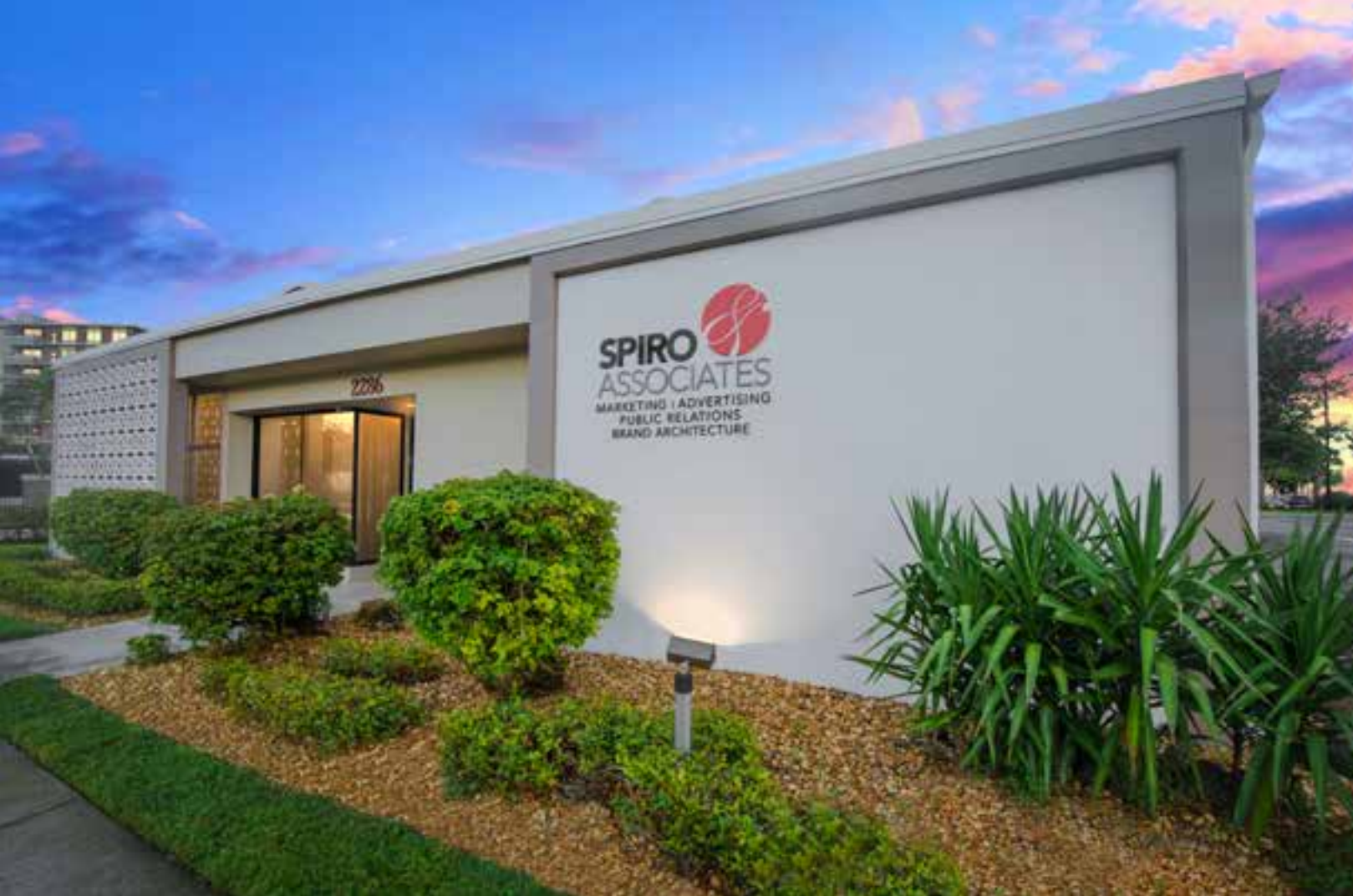
Today – Spiro & Associates' downtown office in Fort Myers, FL.
